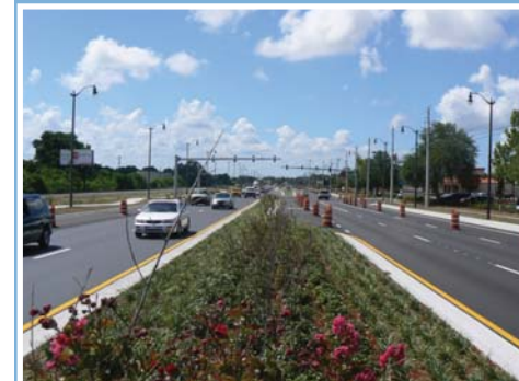
Construction on US 1 from Park Ave. to Pine St. nearly complete
