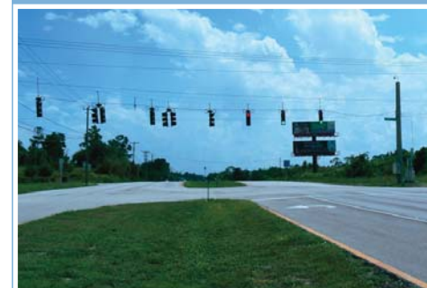
US 1 at Barnes Blvd. before construction
